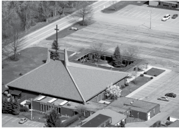
Fig. 2 Aerial view, Saint Jude the Apostle Church (Photo courtesy Robert Tarkowski Photography)
